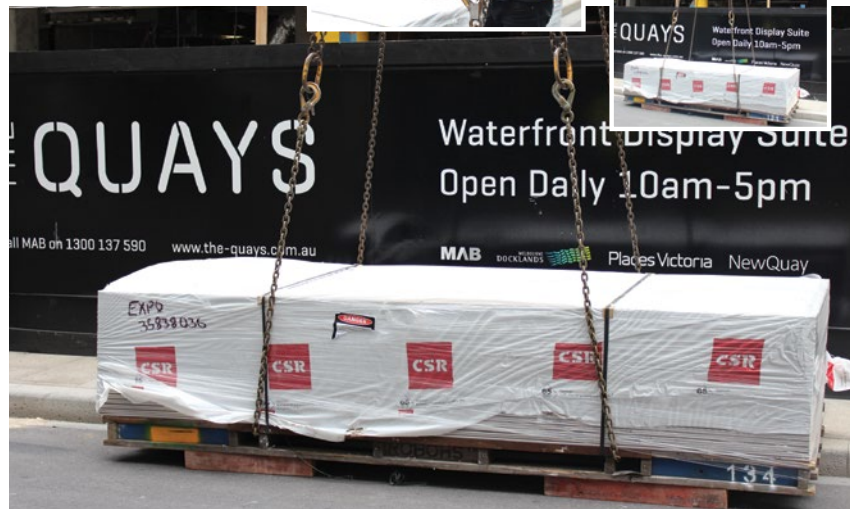
Example of correct use of wrap, strap and ring lifting process, using oblong rings.
